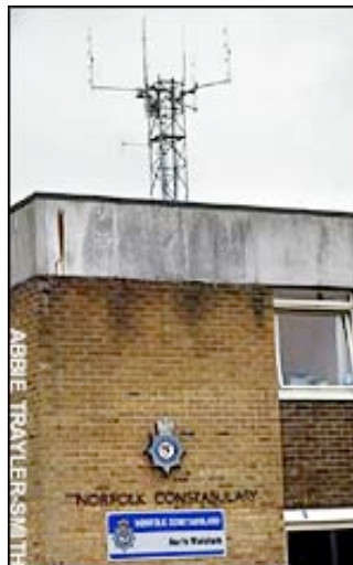
The mast at the North Walsham station
